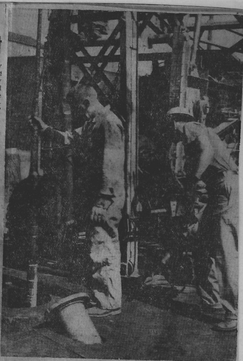
A LONG WAY DOWN —A technician for the Schlumberger Well Surveying company guides an electronic instrument on the first few feet of its 2,260-foot journey down to the bottom of Grinnell's No. 5 well. The instrument determined the type of rock through which the well was drilled.
