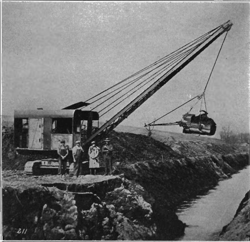
FIG. 25. — Crane equipped with dragline bucket. Courtesy Speeder Machinery Corporation, Cedar Rapids.
