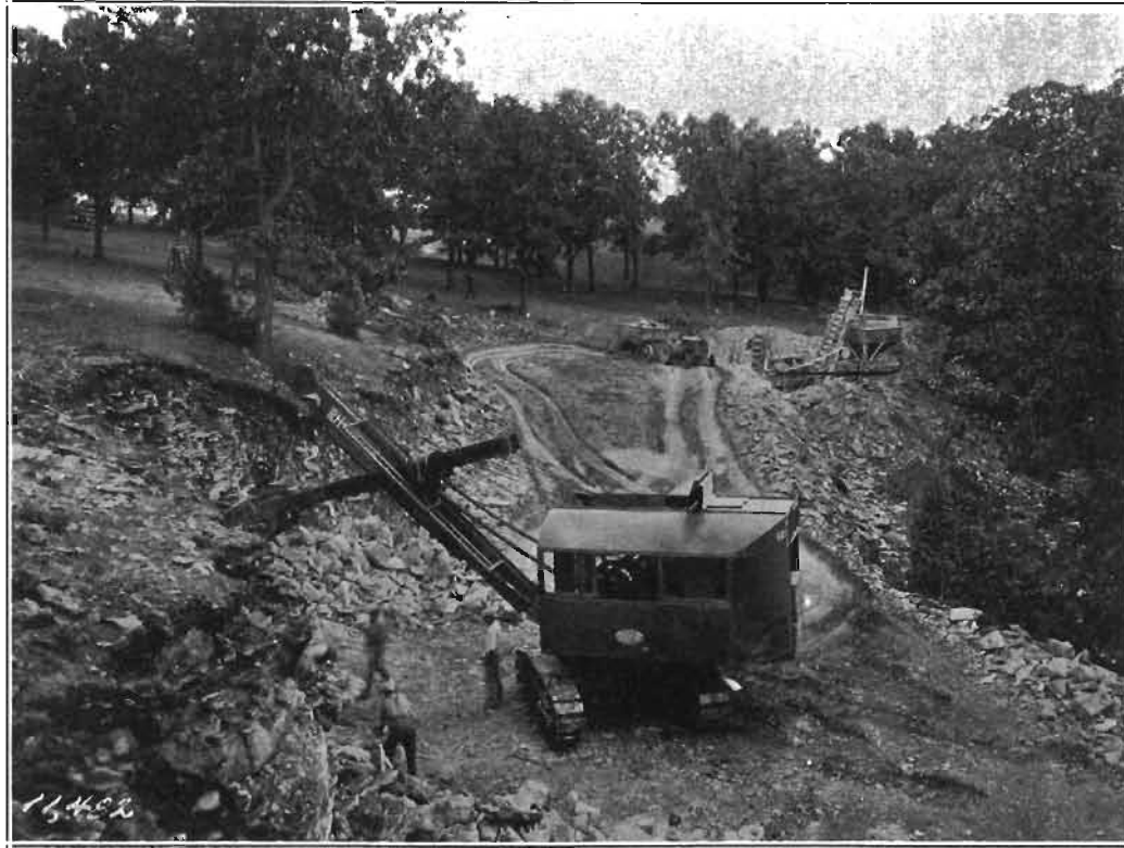
FIG. 34. — Portable surfacing stone plant.
