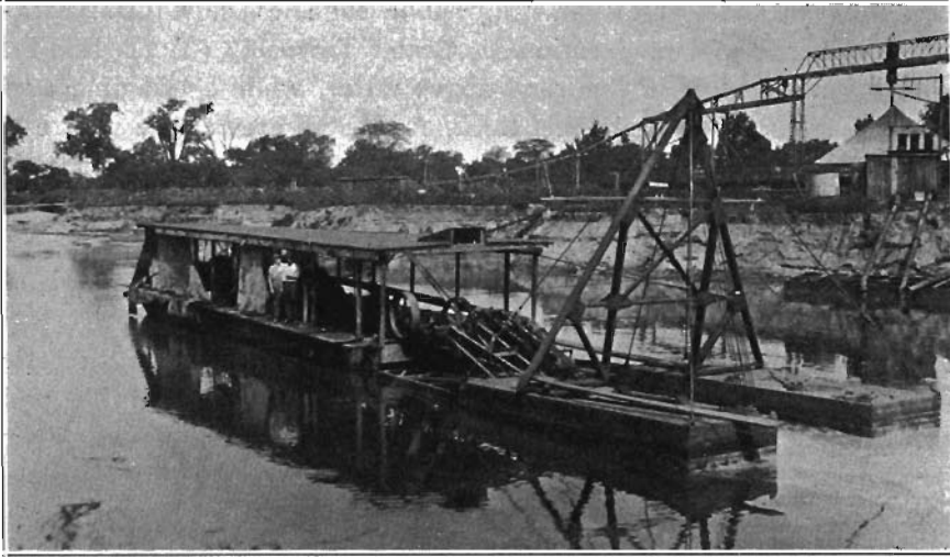
FIG. 14. — Ottumwa Sand Co., Ottumwa. View of Pump Barge.
