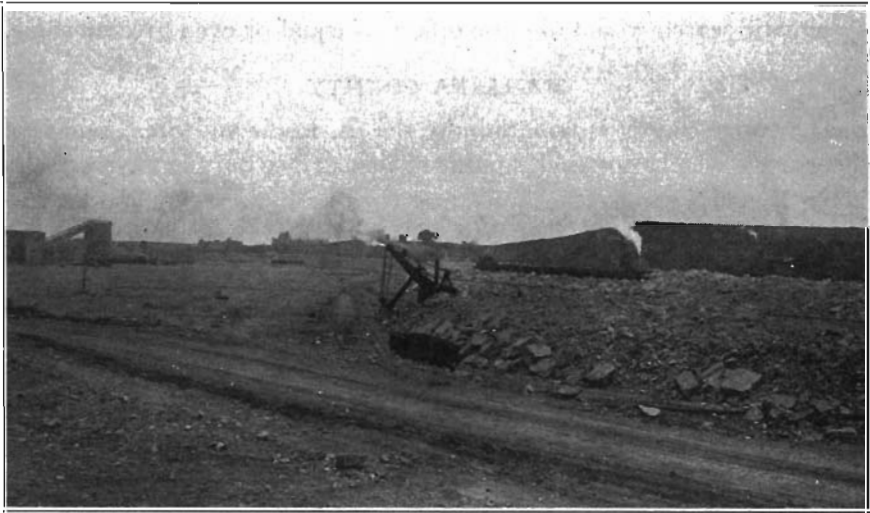
FIG. 5. — General view of Hawkeye Portland Cement Co. quarry at Earlham showing steam shovels working in different quarry lifts.
